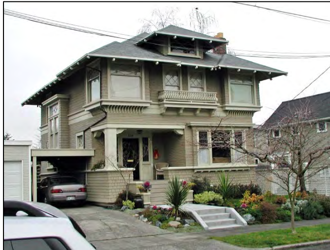
Fig. 56 – Douglas house (1905) at 108 Hayes Street, an example of a “Seattle box.” (DON)
