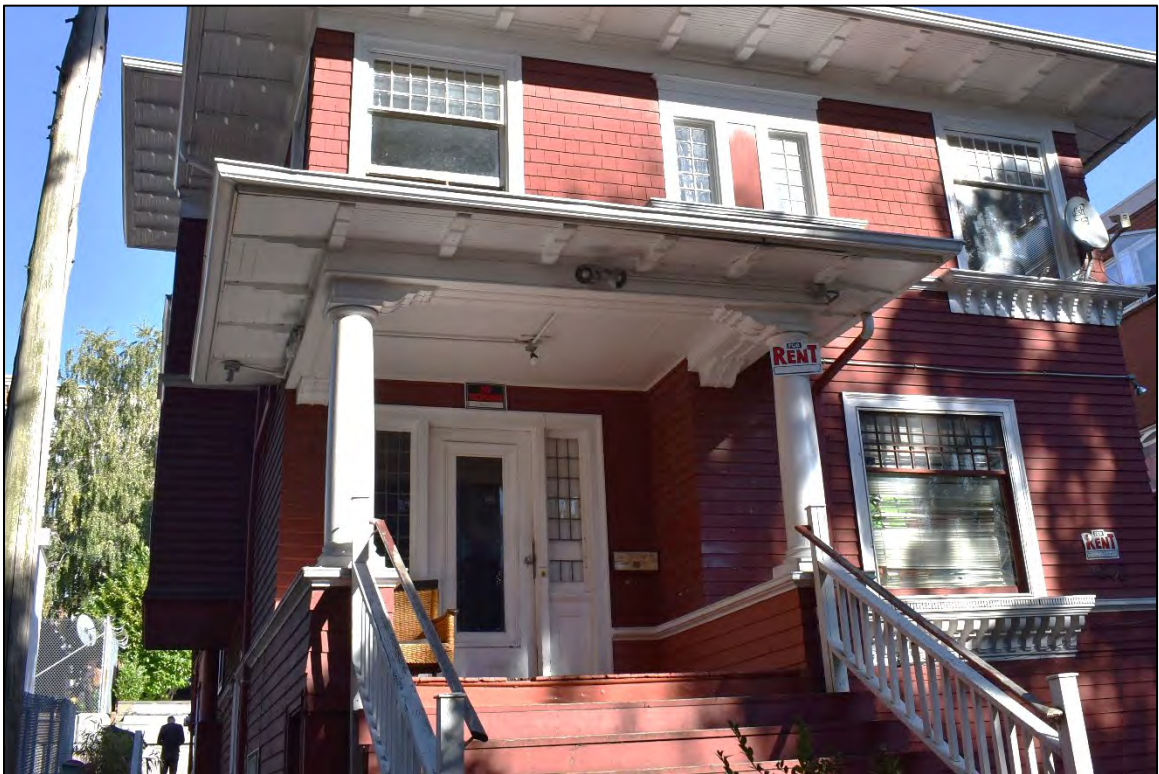
Fig. 8 – West elevation, detail of porch
