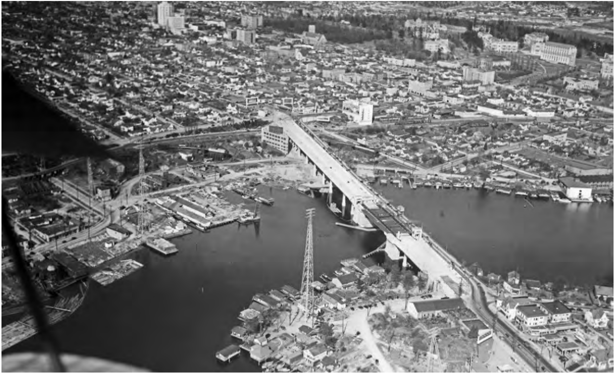
Fig. 43 – 1933 northeastward view of the University District, showing University Bridge in foreground under construction. UW campus at upper right. (SMA 7989)
