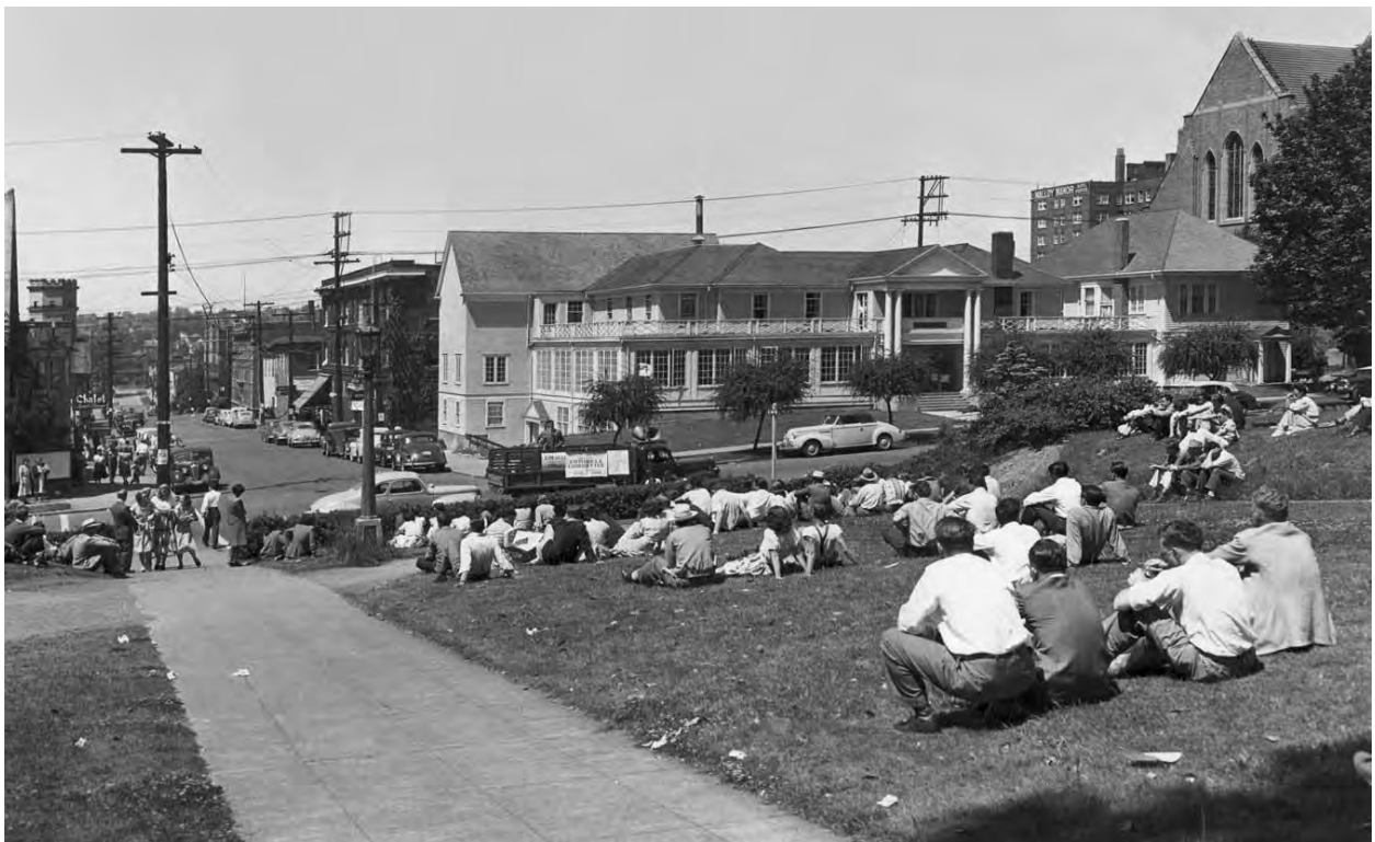
Fig. 42 – 1948 view of 42 nd Street from the UW campus; 15 th Avenue NE crossing in foreground. The tower of the University Methodist Episcopal Church at Brooklyn & 42 nd is visible at far left, one block from the subject site. (Paul Dorpat)
