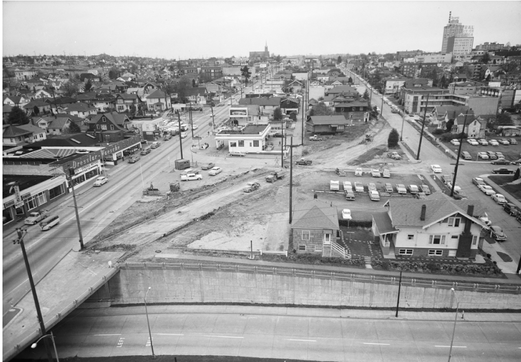
Fig. 48 – 1959 view northward of Roosevelt and 11 th Avenues, being converted to twinned one-way arterials. Campus Parkway in foreground, with retaining wall. Subject property just out of frame near upper right. (SMA #62966)
