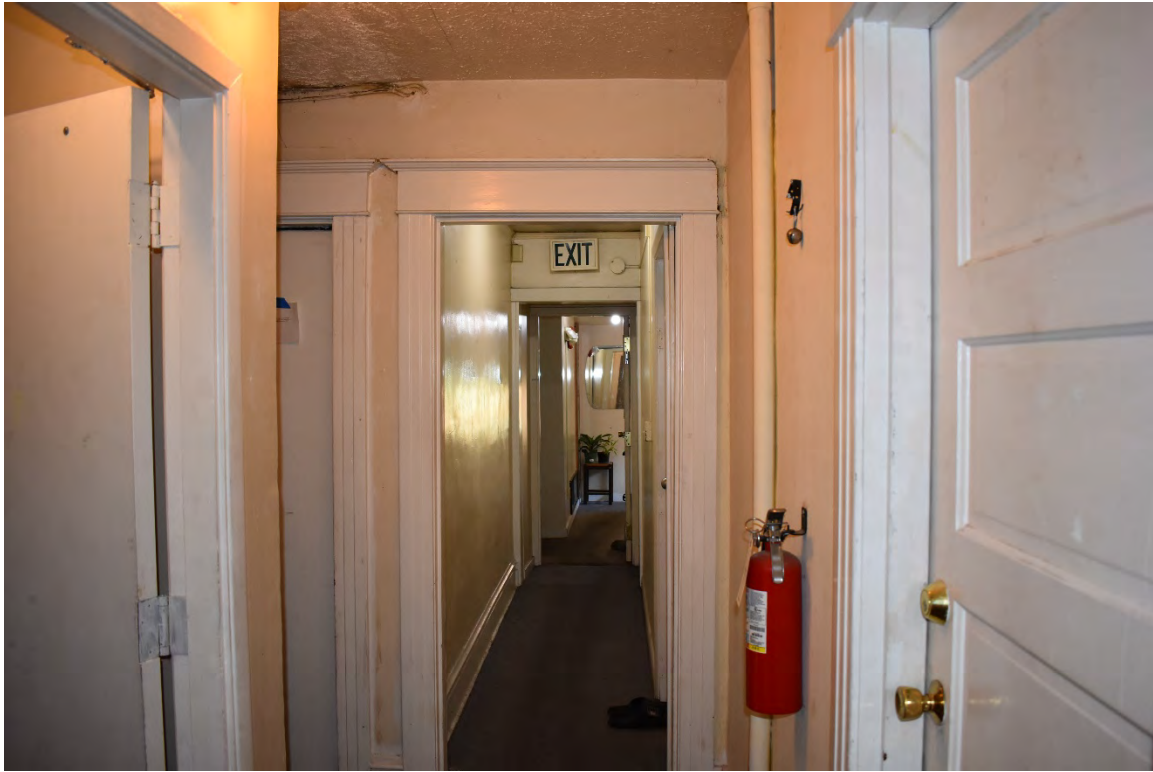
Fig. 17 – Interior, main floor corridor, looking east from entry hall
