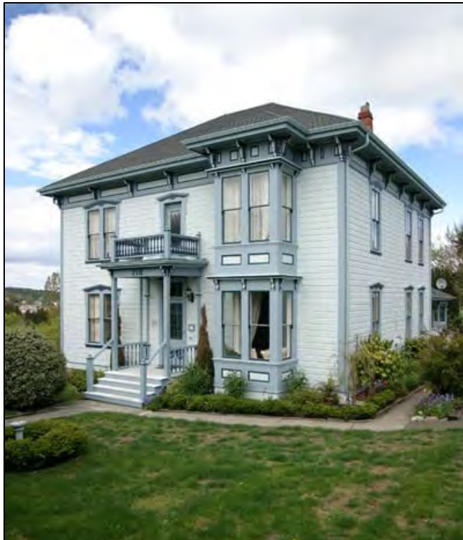
Fig. 51 – Henry Bash house (b. 1885), 718 F Street, Port Townsend, Washington. The house is listed on the National Register of Historic Places.
